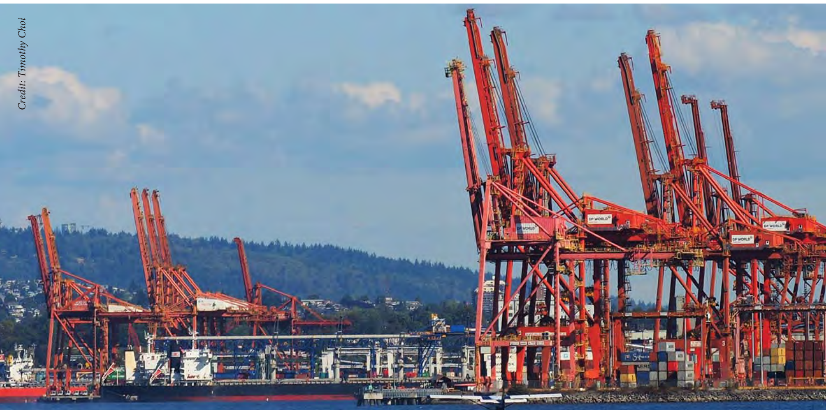
Container cranes overlook Burrard Inlet in Vancouver on 3 September 2018. Despite the immense global infrastructure established to enable maritime trade, much of it is structured around the 'just-enough/just-in-time' mode of supply.
