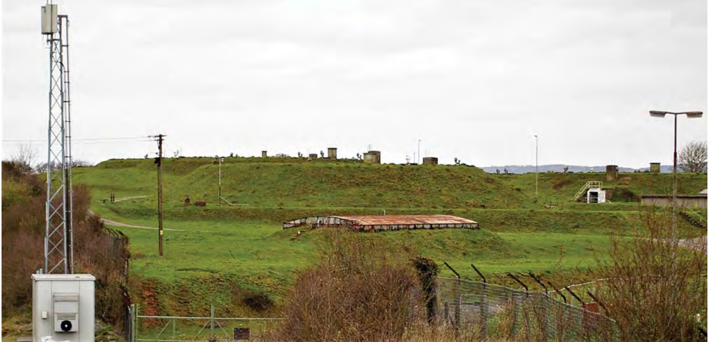
Grass mounds cover fuel tanks at the defunct Flax Bourton underground fuel depot in this March 2014 photo. It was part of the UK's Government Pipelines and Storage System, built to store aviation and other fuels during the Cold War.
