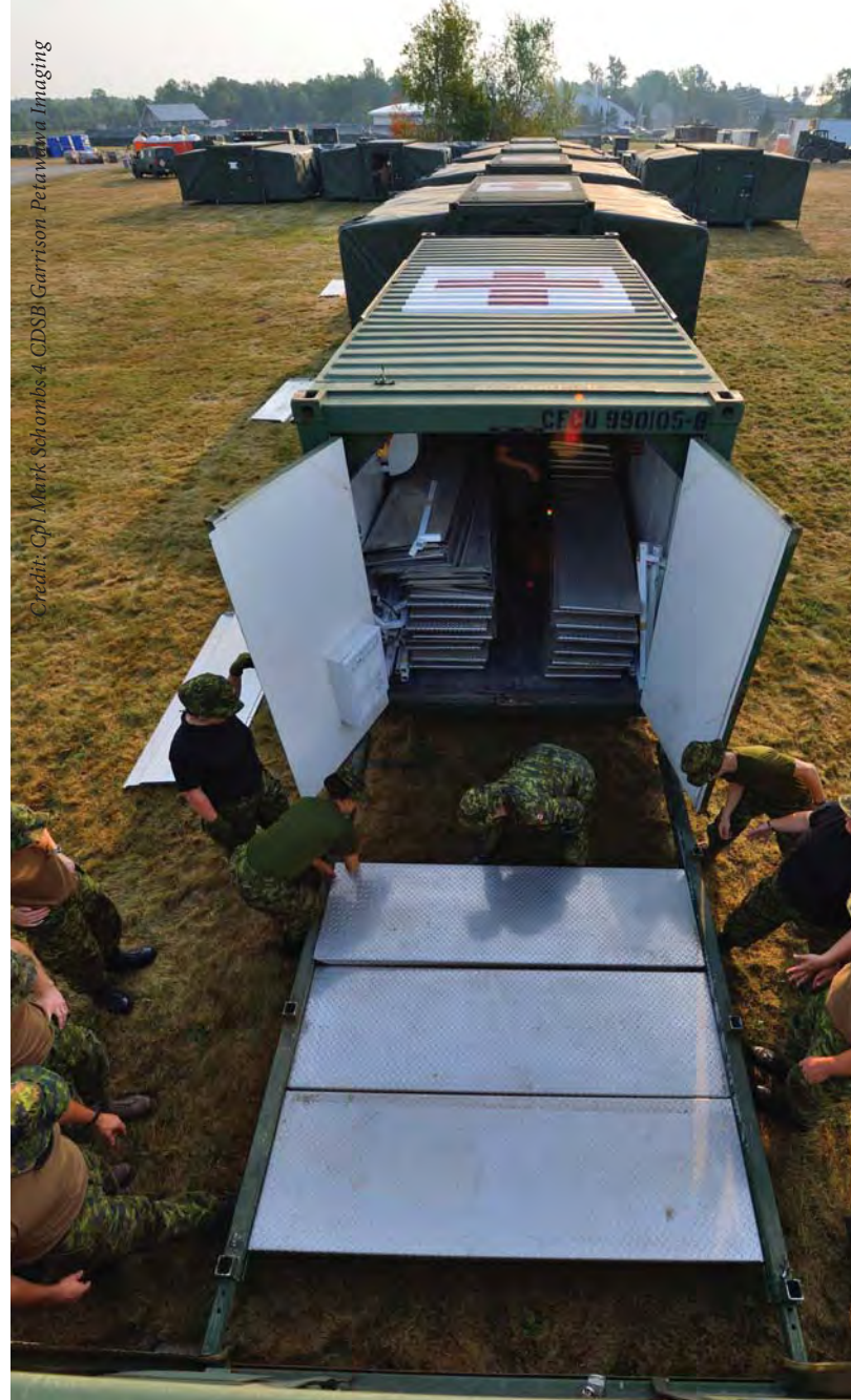
Members of 1 Canadian Field Hospital set up flooring for the Mobile Expandable Container Configuration during Exercise Collaborative Canuk at Canadian Forces Base Kingston on 9 September 2015.
