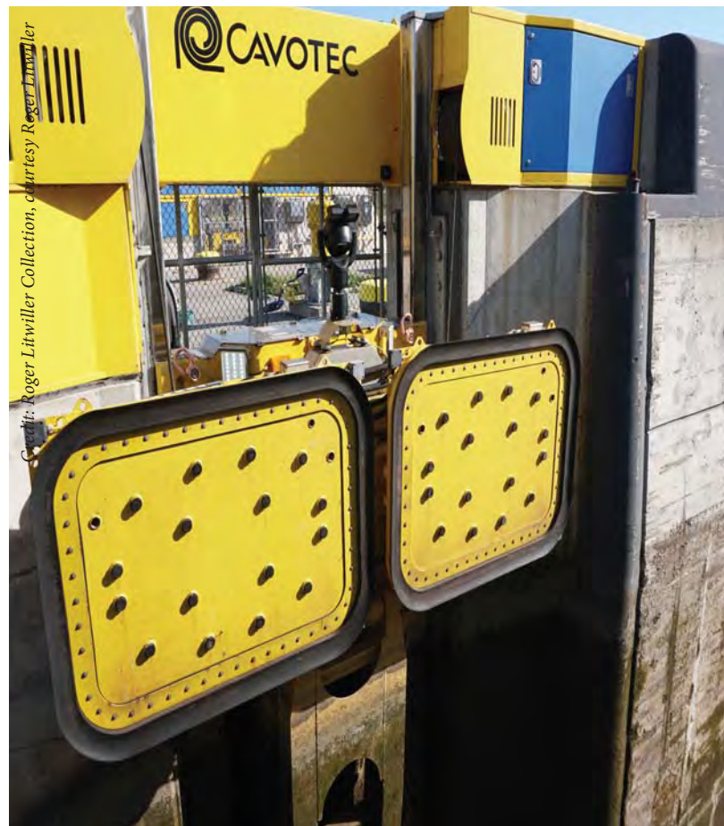
Hands Free Mooring units are installed in Locks 1 to 7. Utilizing suction, these units attach to the ship's hull and hold the vessel securely in the lock, alleviating the time required to secure a ship with lines.
