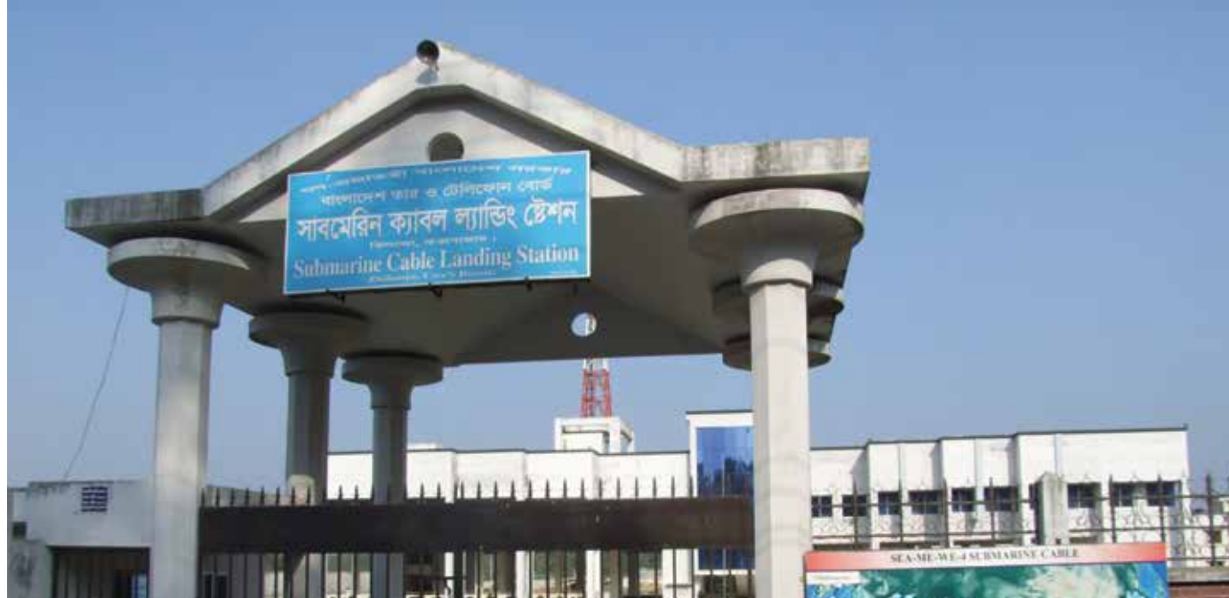
A SEA-WE-ME 4 submarine cable landing station in Bangladesh, January 2006.
