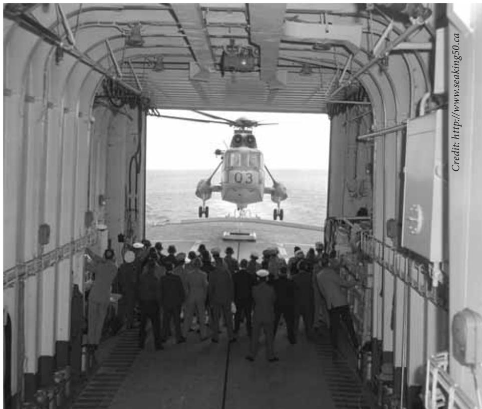
*This photo illustrates early tests of the Helicopter Hauldown and Rapid Securing Device – the innovative Beartrap system.*
